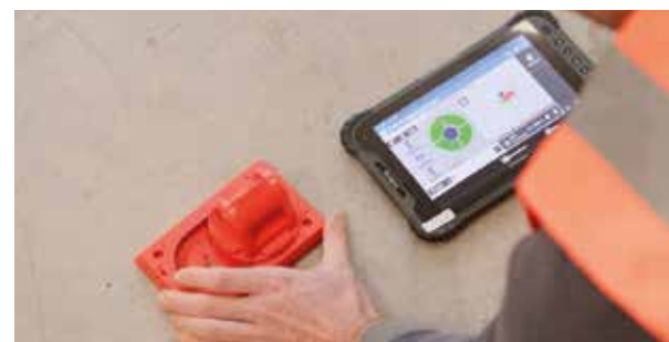
Move the stake out aid on the base plate until the target position is reached – visible on the green circle.
