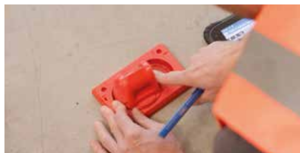
Slide the prism to one side and mark the target position with a pencil.
