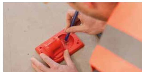
Move the stake out aid on the base plate until the target position is reached – visible on the green circle.
